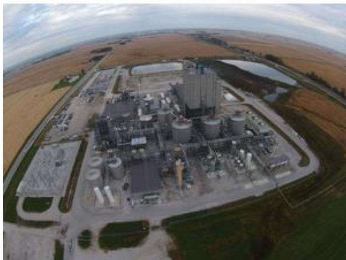
DuPont opens commercial-scale cellulosic ethanol plant in Iowa
