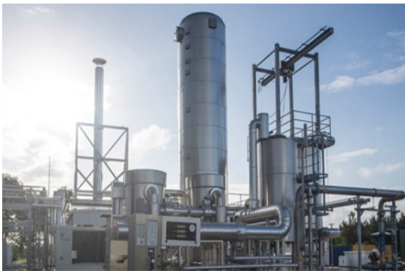
Fig. 3 Power-to-Gas Plant to Produce E-Gas
