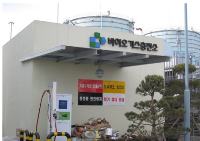
Fig. 3 Biomethane Charging Station
