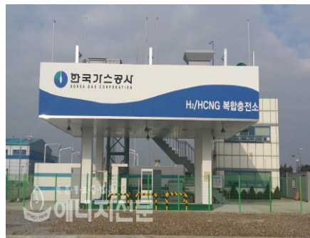
Fig. 2 KOGAS H 2 /HCNG Station
